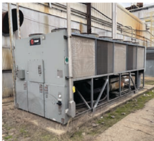
Trane Air-Cooled Series R Chiller
